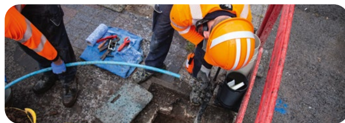
Teams installing a smart meter, Coventry
